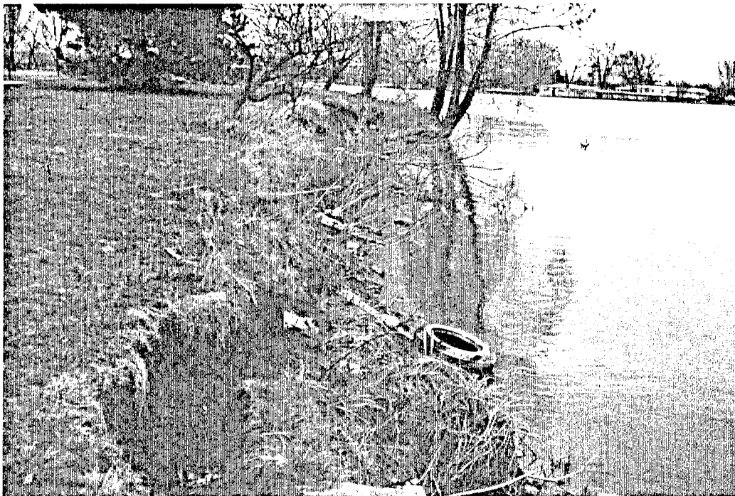
14. Looking east along north shore of lake. Active erosion. Not critical but loss of land base is occurring.
