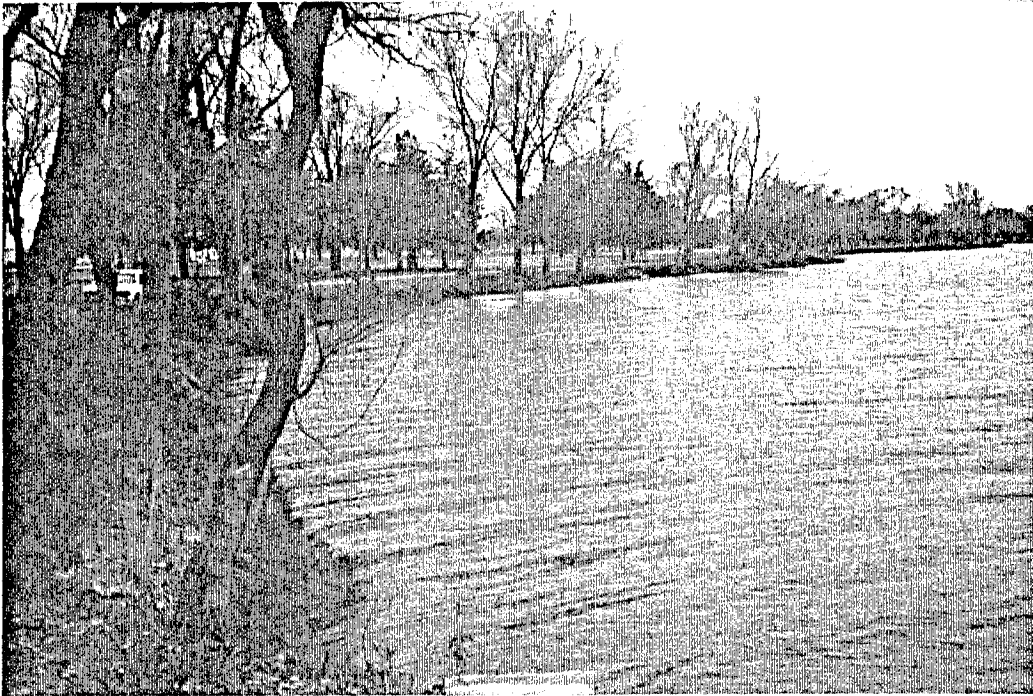
13. Looking southerly along east leg of lake. Some erosion along trees and access road.
