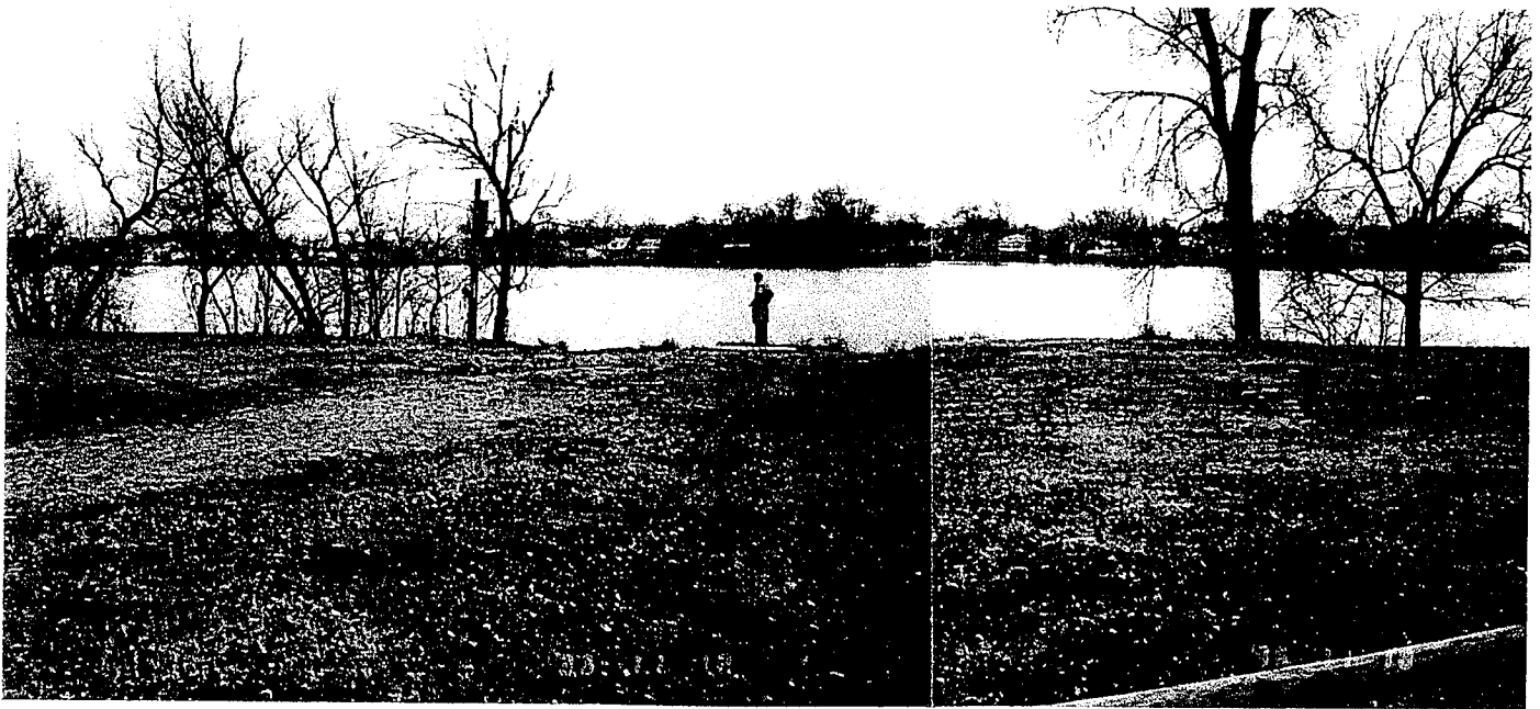
View looking southwest toward the proposed wet well location at the edge of Carter Lake.
